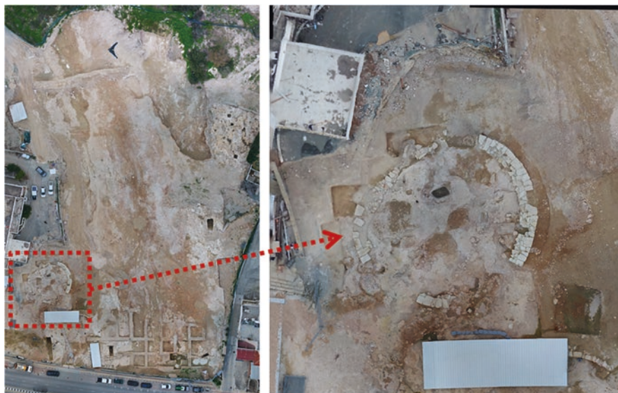
Fig. 31 Ortho-image of the overall excavation site in Amathus, including detail of burial site
