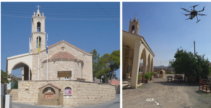
Fig. 18 Foinikaria church, with UAV flyover and ground control point (GCP)
